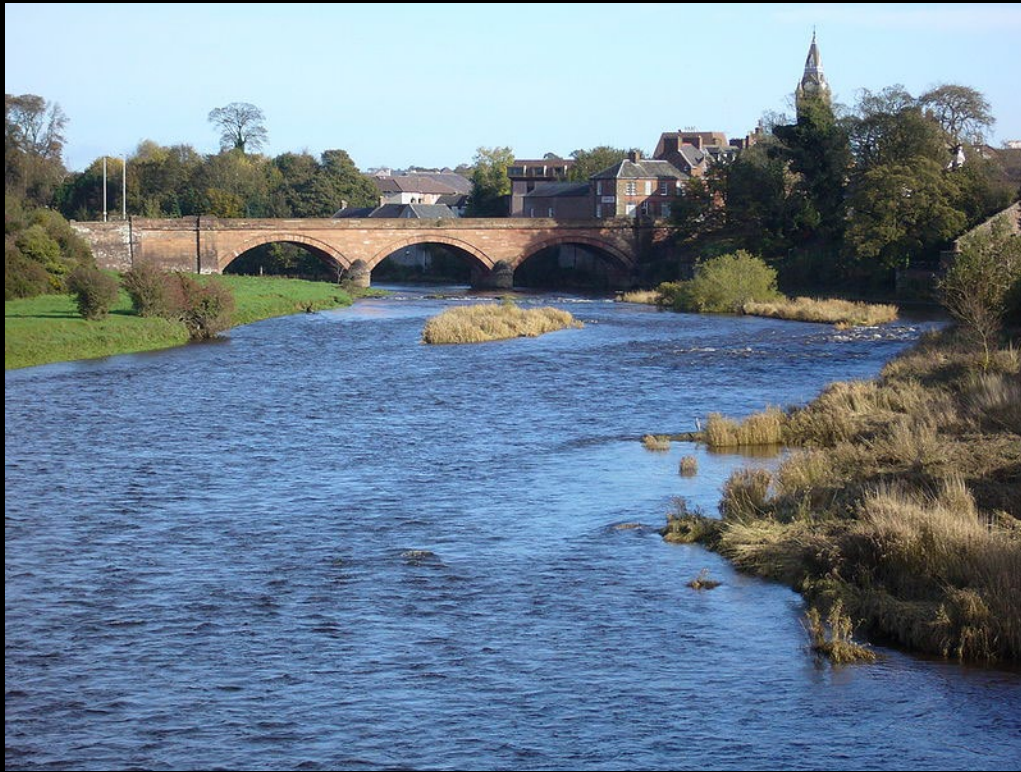
The Annan River Bridge
